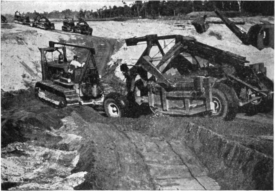
Figure 130. Earth-moving equipment operating in a select-material pit.
